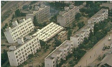
Example of Damage from Soil Liquefaction
