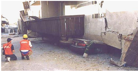
Building failure due to soft story condition caused by tuck-under parking
